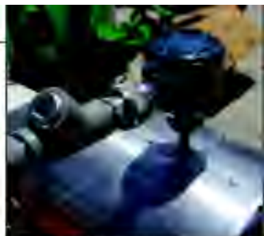
FIGURE 4. A temperature transmitter is a rugged, field-mounted device that can be installed directly on the sensor and thermowell.
